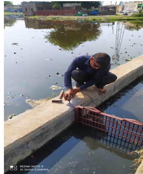
MESH INSTALLATION AT INLETS
